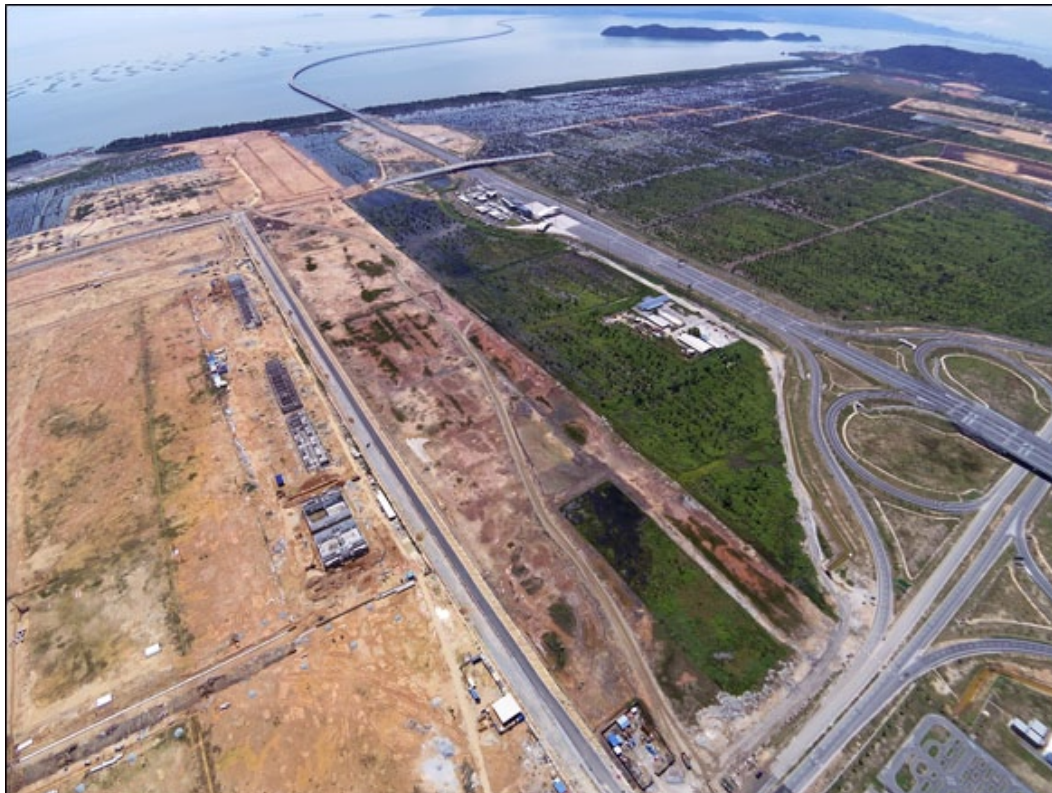
The landing site of the Second Penang Bridge at Batu Kawan.
